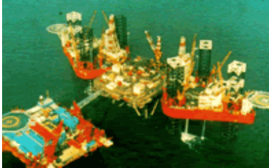
Morecombe Bay Gas Platform
